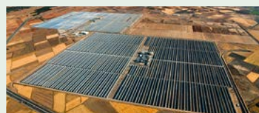
The Andasol solar power station
