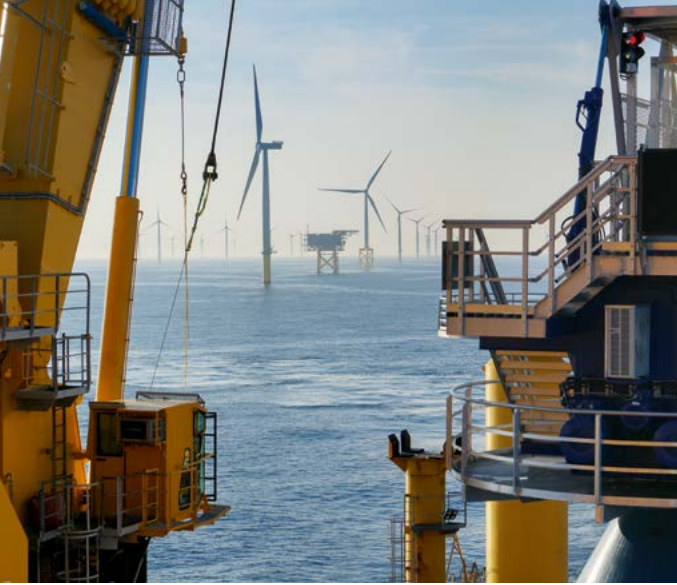
A view from the substation of the wind turbines of the “Borkum Riffgrund” offshore wind farm – and the “endless” expanse of the North Sea
